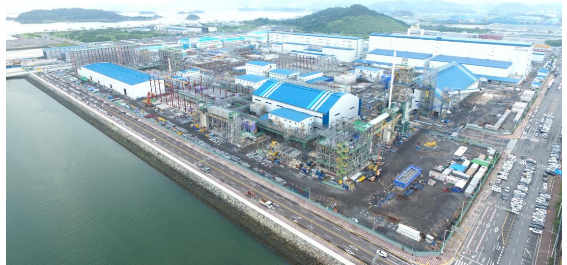
August 2023 Construction site at the POSCO Pilbara Lithium Solutions LHM facility
