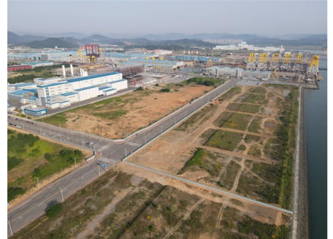
May 2021 Breaking ground
