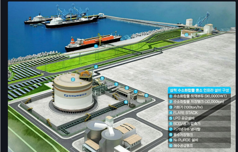
A rendering of Samsung C&T's forthcoming ammonia-handling infrastructure at the Samcheok coal plant. (Photo: Samsung C&T)
